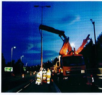
Mallatite has supplied aluminium lighting columns and LED road lanterns as part of the Erskine Bridge Lighting and Electrical Refurbishment Project for Transport Scotland. The project is set to enhance night-time driving visibility and also reduce energy usage by 70 to 80% with dimming. The A898 Erskine Bridge is a large
